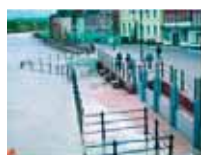
Demountable Flood Barrier
