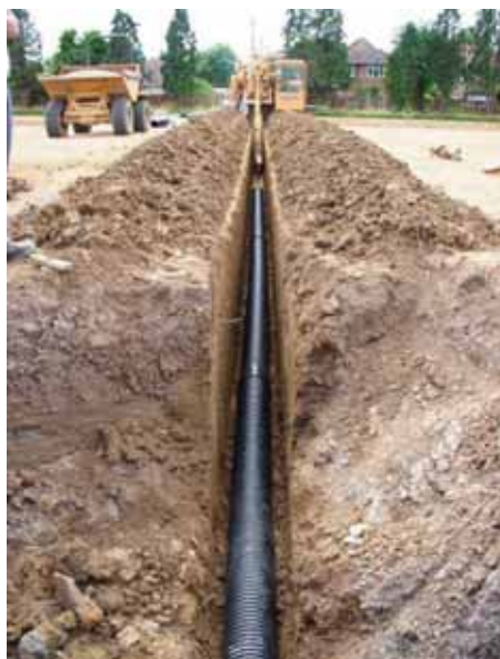
Land drainage pipes being installed and even the turfgrass for your local sports club, golf course, or the park where you take the kids to play and walk the dog on a Sunday morning.
