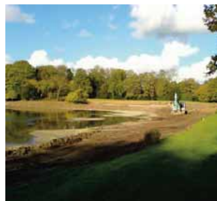
A lake under construction which catches and holds water reducing flooding downstream
