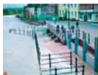
Demountable Flood Barrier
