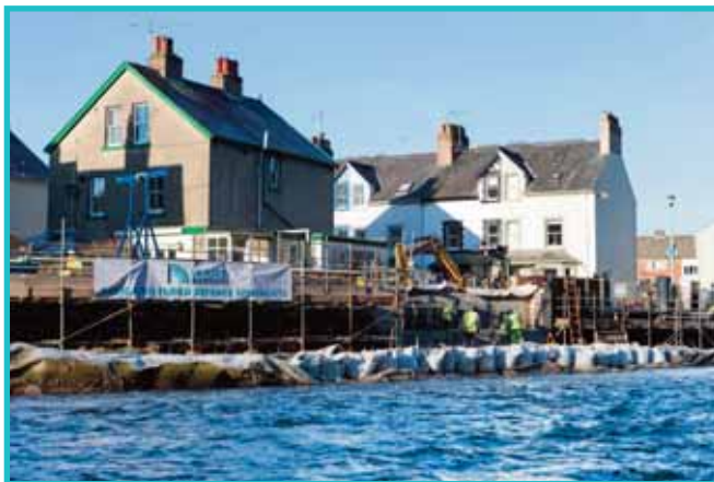
Left: The UKFB installation team on site.
