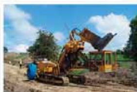
Other Drainage Works
