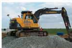
Utility Installation &amp; Trenching Works
