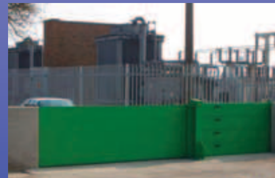
Combination flood gate/ demountable barrier to wide vehicle access
