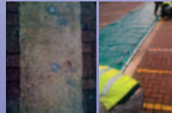
For known locations a concrete beam is fixed into position for the RapiDam Bolt Down system to be secured to
