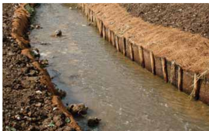
re-profiled banks with brush bundles and coir rolls
