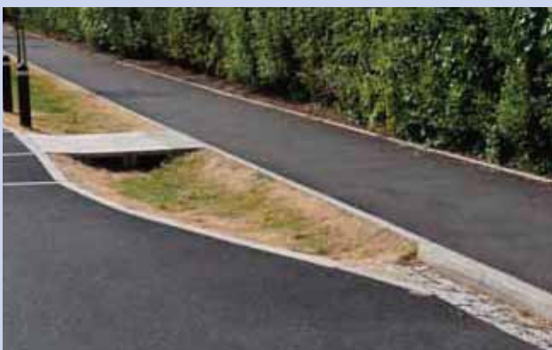
Bullnose kerbs to the road and edgings to the footpath allow runoff to flow gently into a swale without erosion. A simple pedestrian crossing is formed with concrete paving flags.
