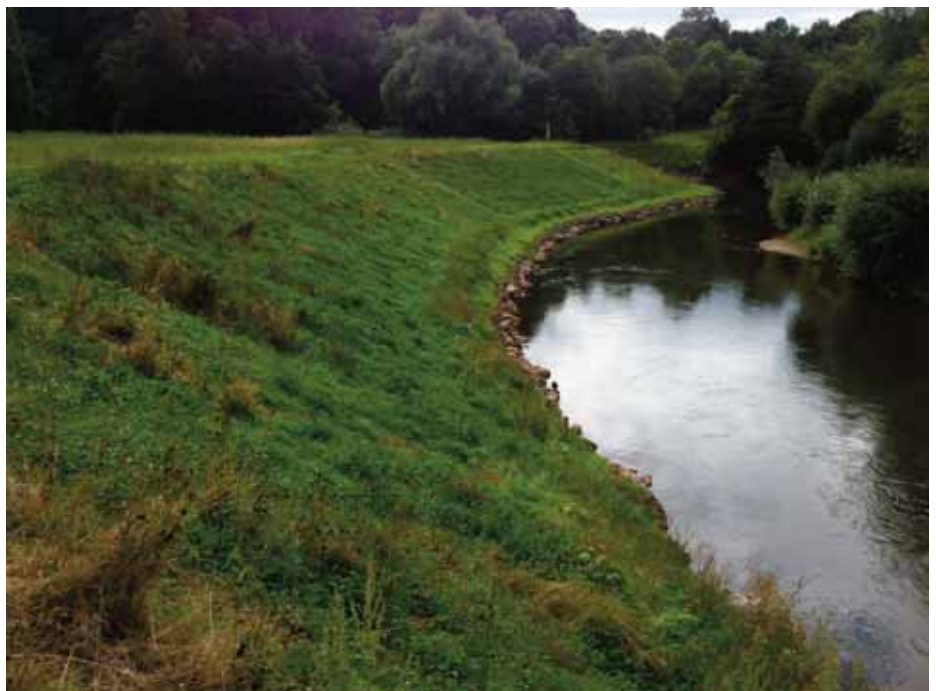
Post floods and two months after the end of the works, the River Teme is free from the ravages of erosion.
