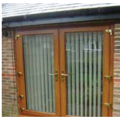
Double Flood Angel® Flood Defender™ Doors installed to the rear of a property
