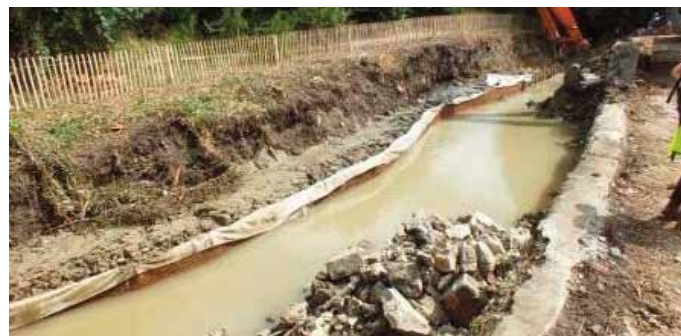
The far bank coir revetment being installed
