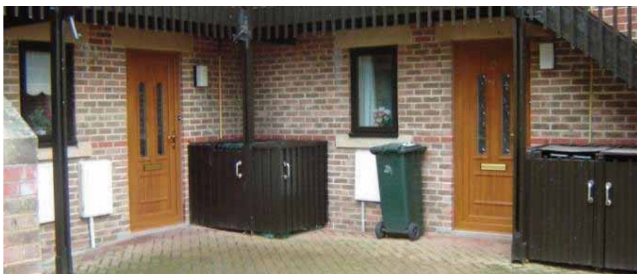
A total of 31 Flood Angel® Flood Defender™ Doors were installed for this project
