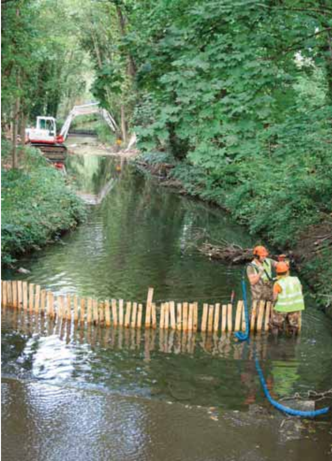
The upper line of posts going in with the weir being removed in the background
