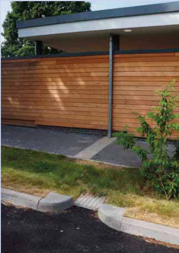
Kerb quadrants direct water straight off the impermeable access road into a swale, softened by a concrete flag. Rainwater downpipes from the building roof discharge directly over ribbed concrete flags which channel the water across a footway.
