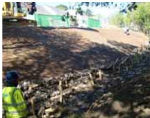
rock rolls in place protecting the toe
