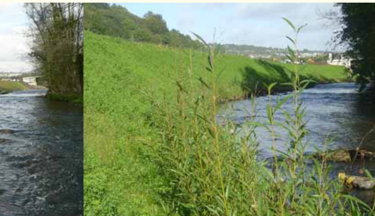
left: River Ebbw, with Tensar VMax P550 erosion control installed right: River Ebbw one year after erosion control and greening
