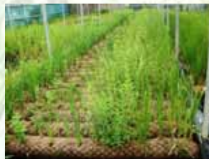
Vertical Bank Revetment with pre established coir rolls
