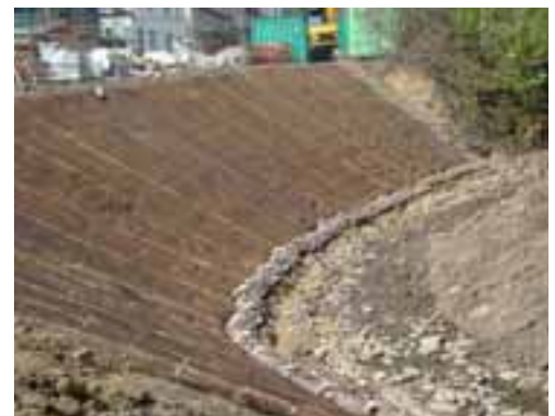
the graded bank, covered with the VMax C350
