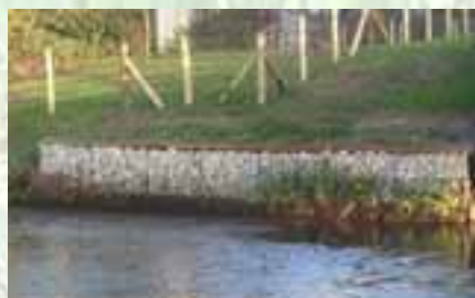
Hard & Soft Engineering Solutions - coir fibre edge sods used to soften up a gabion retaining wall
