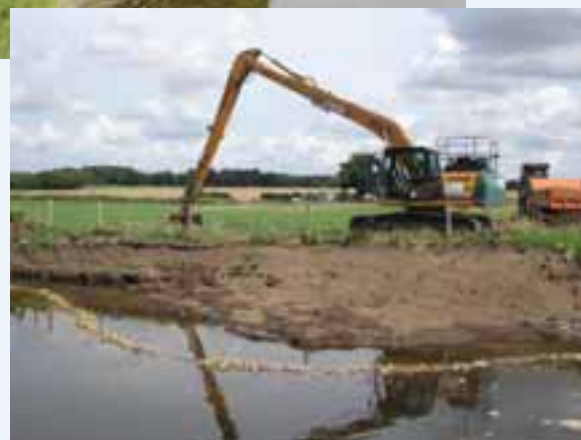
above: Bed raising using gravel to create glide. In total 6 glides have been installed along the 800m length of river being restored.
