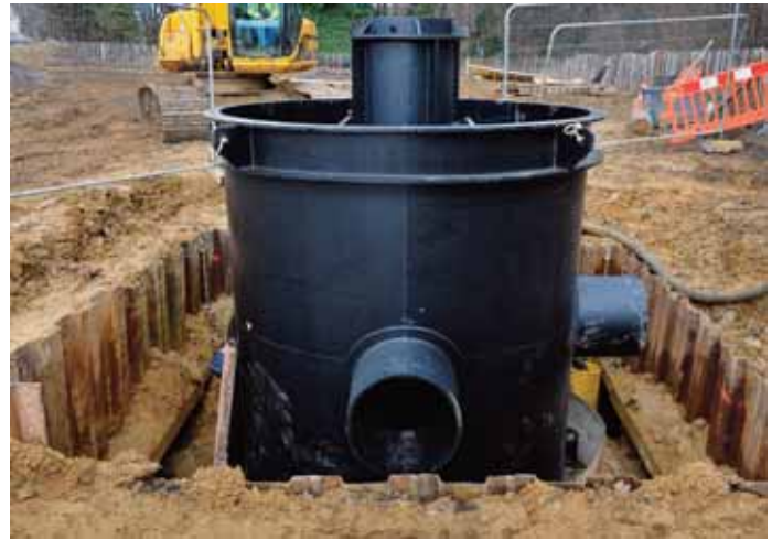
Installing a Downstream Defender ®
