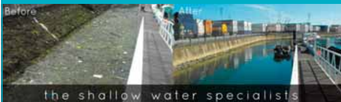
River Dulais demonstration project using live willow root wads revetment techniques in place of blockstone
