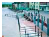
Demountable Flood Barrier
